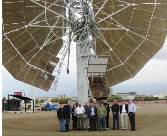
Conference attendees stand at the base of Southwest Solar Technologies' 22 meter, multiple mirror panel parabolic reflector. The reflector is pointed toward the ground and the square white screen on the boom just above the group was installed at the focal point for astronomical observations that night. Sadly, it remained cloudy so we were unable to make the observations, although we enjoyed our extended dinner ☺.
